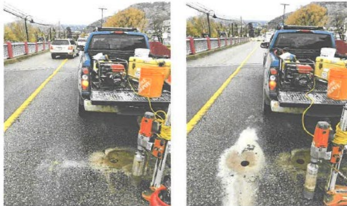
Photos 3 and 4 – East approach to the bridge (±10m east of bridge)
